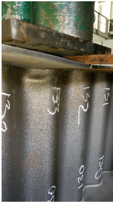
Fig. 7. Local buckling of the corrugation
